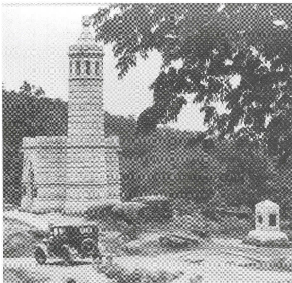
Figure 18. The South Loop of Sykes Avenue, Little Round Top, c. 1930. This was the southern of two loop overlooks atop Little Round Top constructed in 1897. It took visitors to the castle monument placed by the 44th and 12th New York Infantry veterans and afforded visitors an excellent view of Devil's Den and the Valley of Death from their carriage or vehicle. The GNPC constructed new telford roads, bridges, and retaining walls throughout the park to give visitors easy access to all key battlefield sites. Park road construction began in 1894 and heightened the popularity of the Round Tops, Seminary Ridge, and other rough terrain spots in the park considerably (ACHS).
