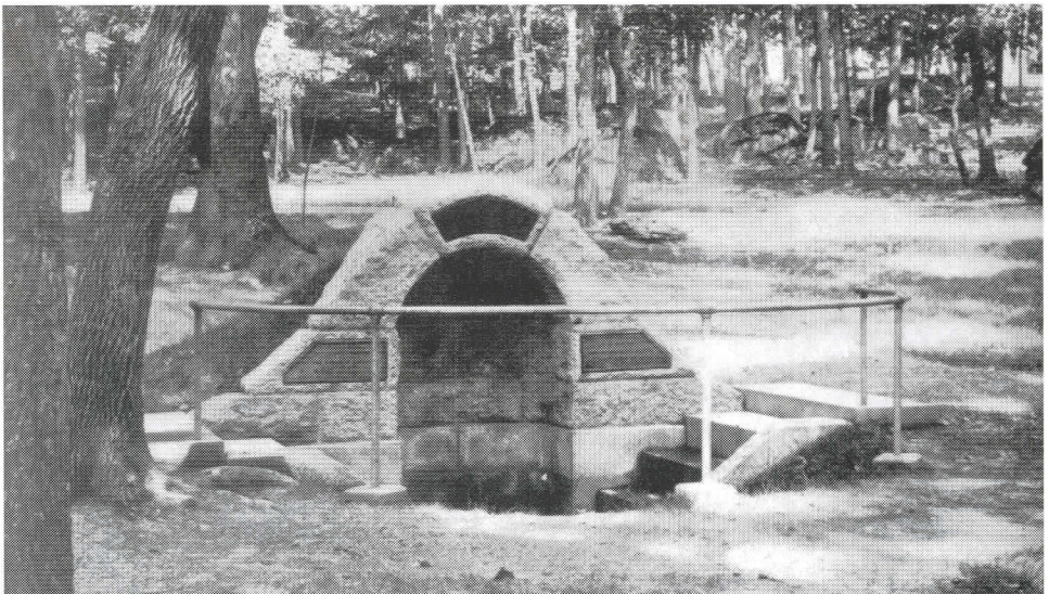
Figure 2. Spangler's Spring, 1900. Originally, there were two stone outlets for the spring here. After 1895, the War Department ordered the GNMP to tidy up the field and Spangler's Spring received a makeover. The cement half-dome, steps, and rail are entirely new (GNPC, Annual Reports).
