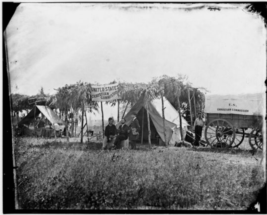
USCC headquarters in Germantown, VA. Photo via Library of Congress.
