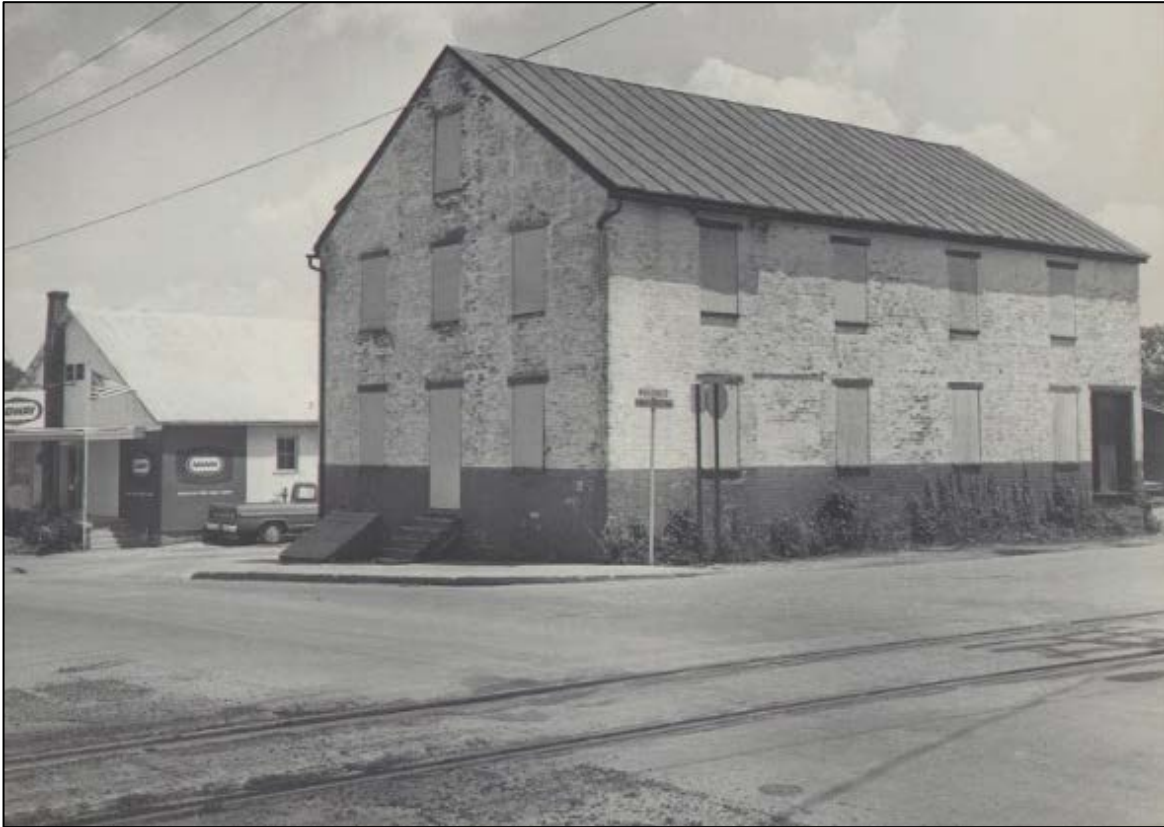
Figures 7-8. Then and now comparison at the site of the North Washington Street Freight Station. Historic photograph courtesy of the ACHS.
