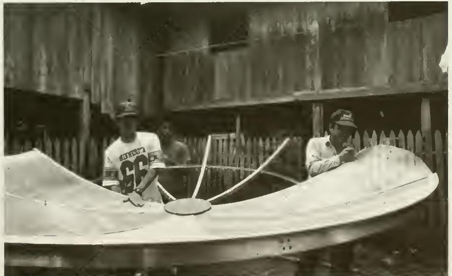
Fig. 9. Assembling a satellite dish.
