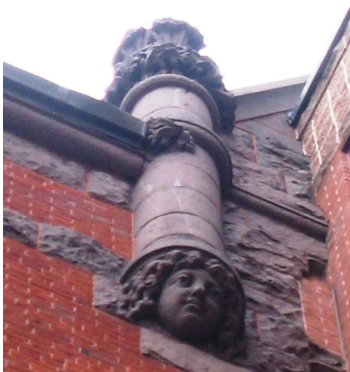
Tower Beside Elevator Addition
