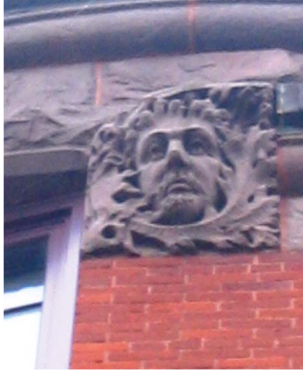
West Front Parapet
