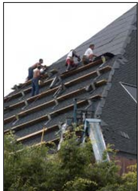
Musselman Library gets a new roof. Photo by Bill Dowling
