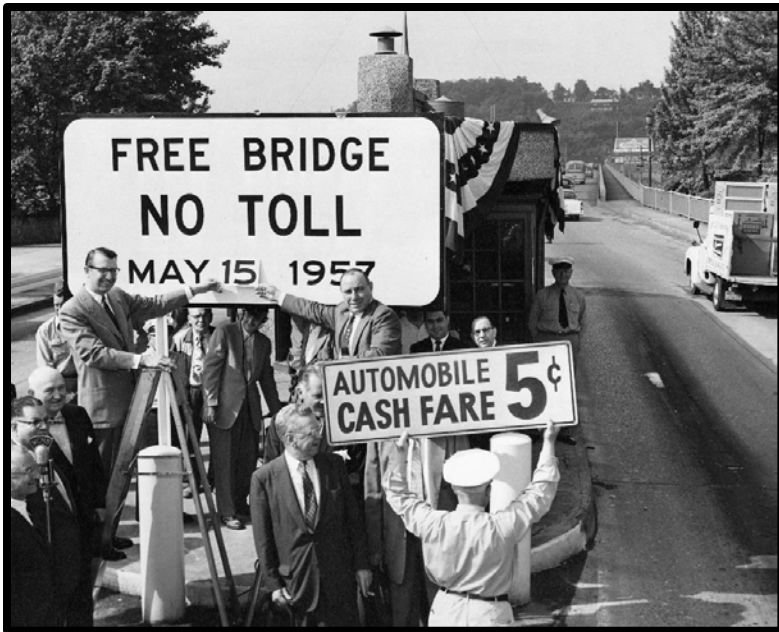
The removal of toll booths from one of two bridges spanning the Susquehanna River between Harrisburg and Lemoyne, May 15, 1957.
