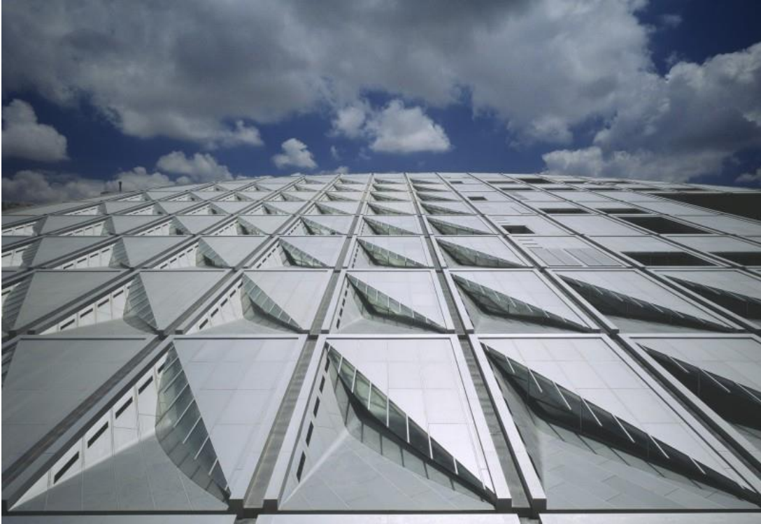
Figure 4. Vertical and north-facing slits in the roof
