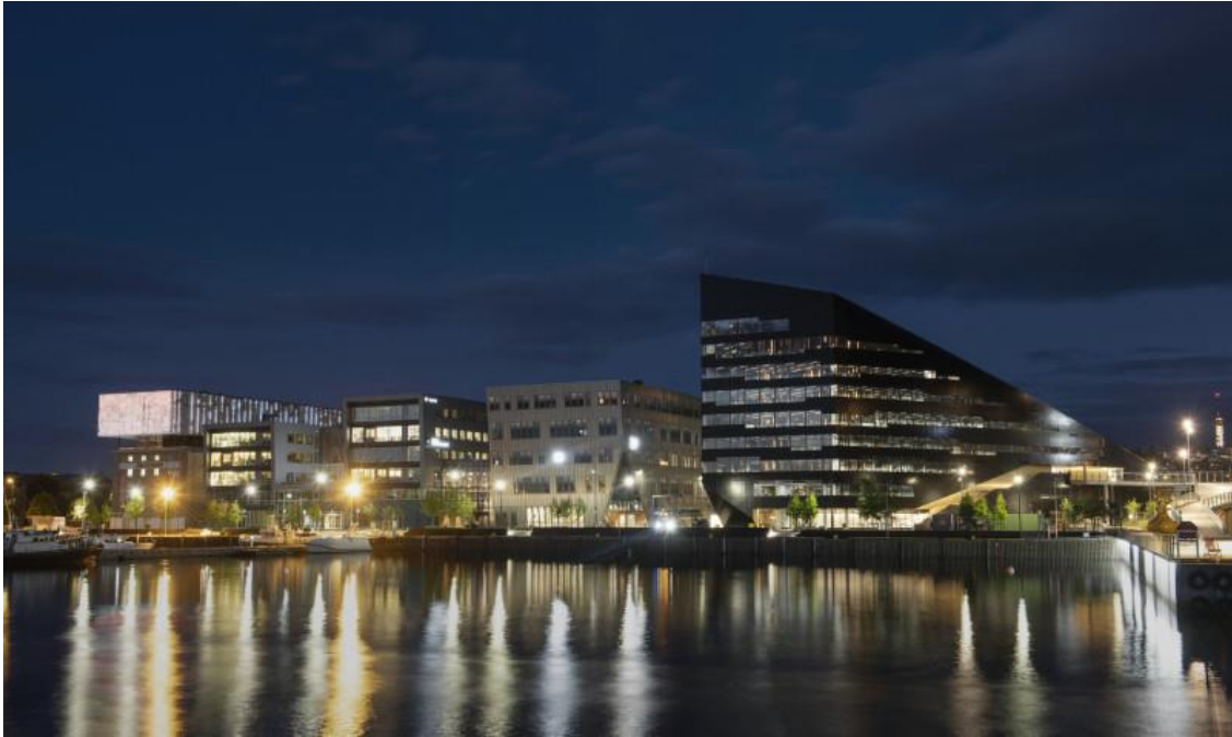
Figure 17. Powerhouse Brattørkaia stands on the right, showcasing how the height of the building is similar to the rest of the skyline
